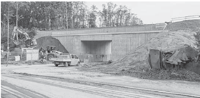
Neue Brücke in Dalheim
